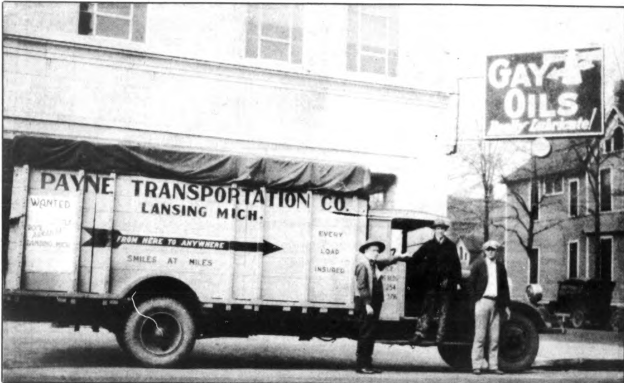
TOP LEFT — During the early decades of the century, this is how Earl Payne hauled gravel.
