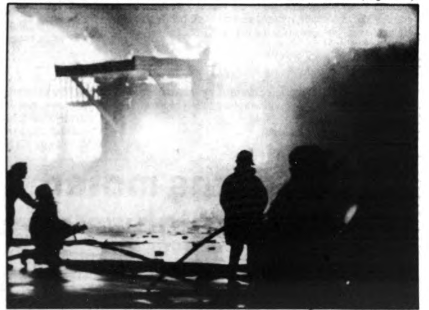
CCN file photograph MAJOR FIRE — The fire which destroyed the Clinton Home Center building in St. Johns was the biggest blaze in St. Johns since the Steel Hotel burned.
