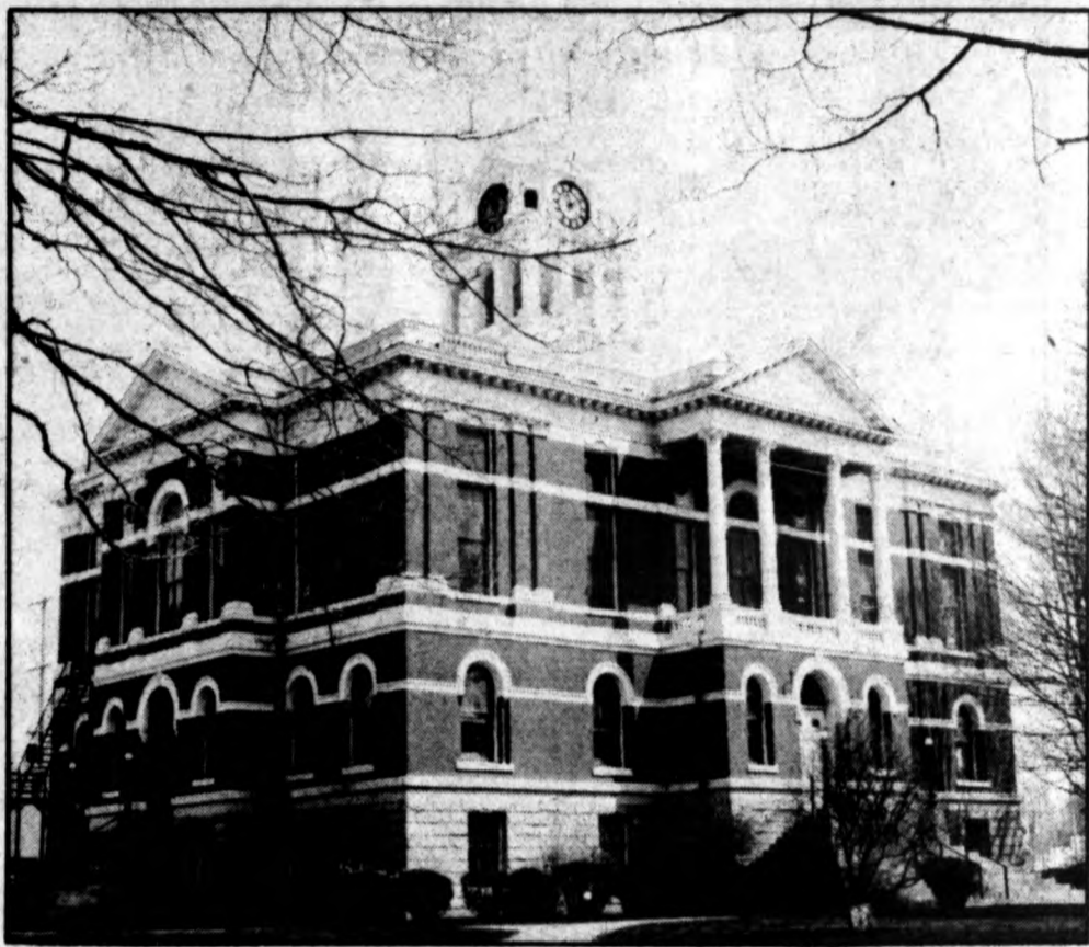
The 1884 Courthouse, a 3½-story building made of fieldstone, red brick and white stone, cost $75,000 to construct.
