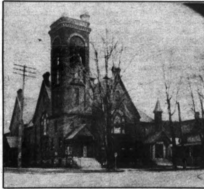
SECOND METHODIST CHURCH This church was St. Johns' second Methodist church, the first being made of wood. It stood at the corner of State and Linden and burned down in 1936.
