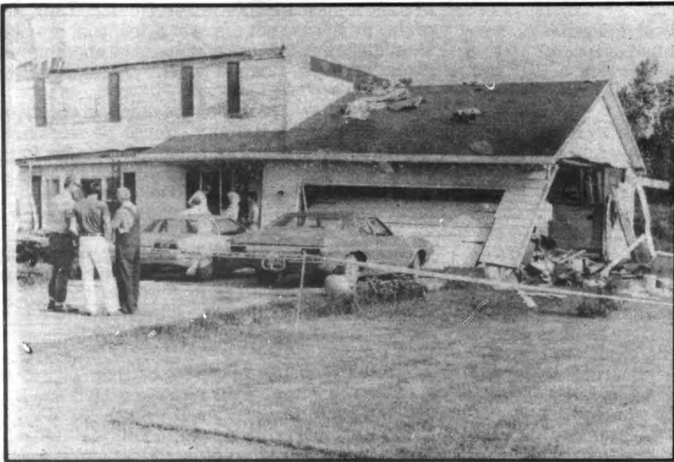
AN APPARENT TORNADO SKIPPED THROUGH THE COUNTY Thursday morning, leaving one couple homeless. Bruce and Rose Welton, of 3176 E. French Road, were preparing breakfast when the incident occurred. Their roof, shown above, was thrown approximately 500 feet from the home, while the foundation of the home was shifted several feet.
