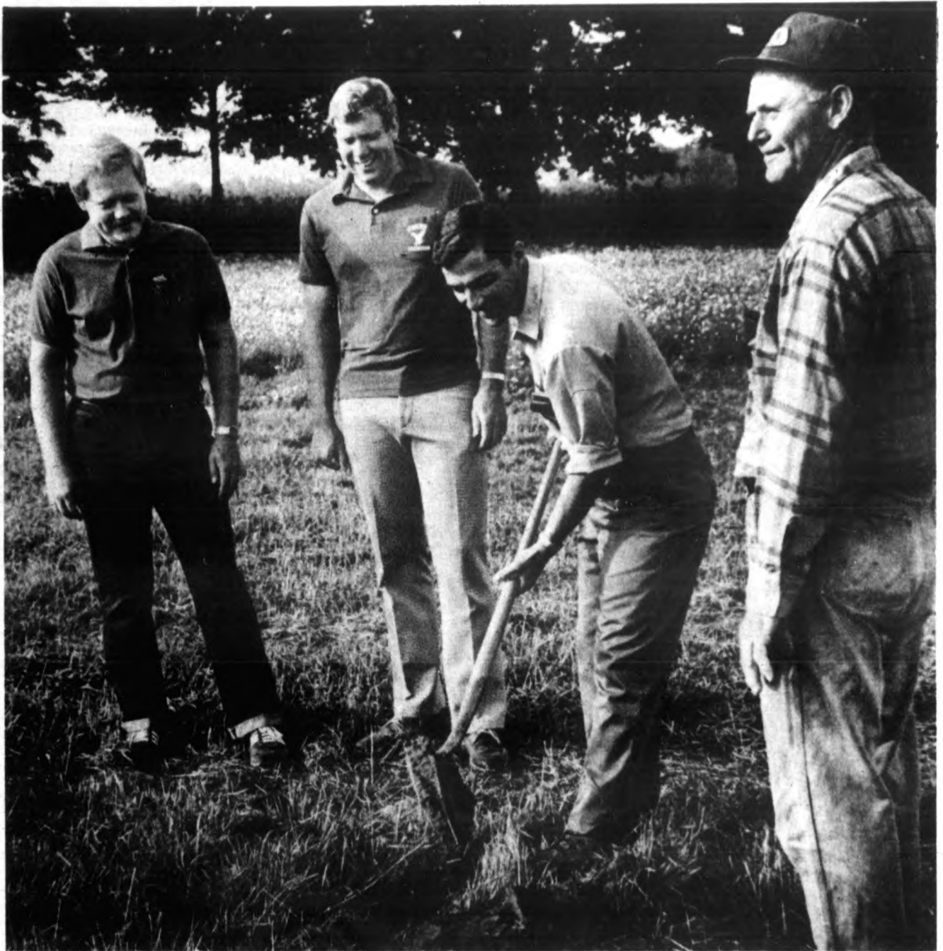
Victor Township Supervisor Robert Remus (with shovel) breaks ground for the volunteer-built Victor Township Hall. Watching the
