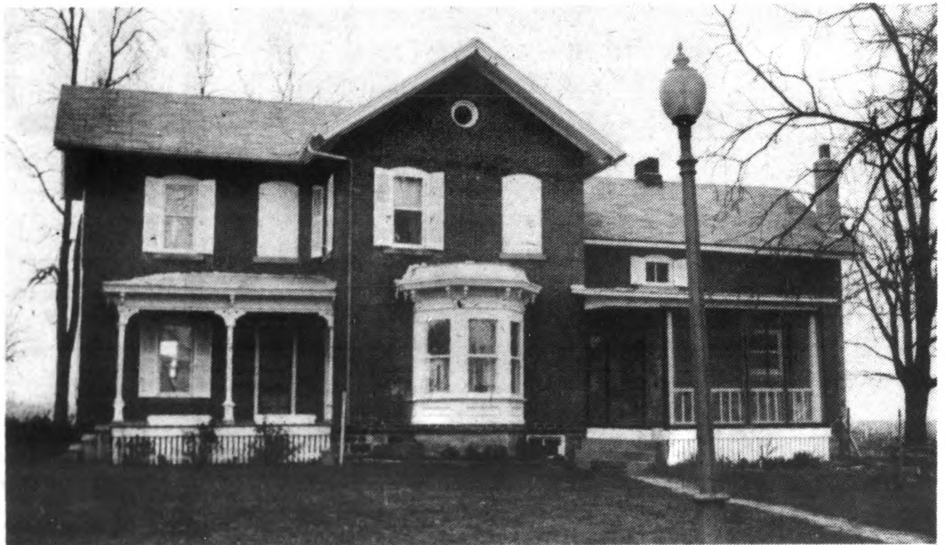
This brick farm house on Francis Road in Watertown Township is very similar to many of Moon's other farm houses which he designed in Eaton County. Built in 1878 for Willard King, it is now own-
