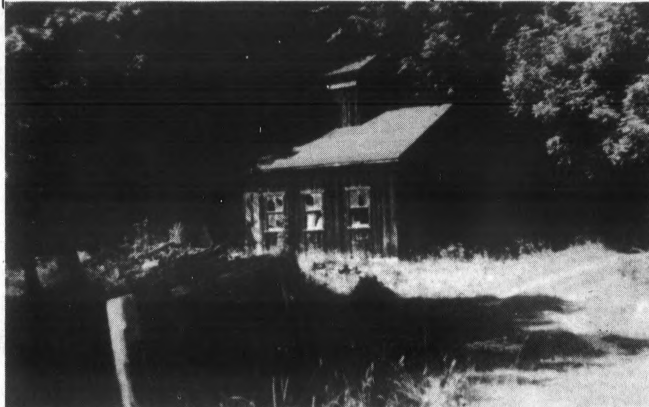
The final photo in our presentation of Clinton County's prize winning entries in Eastman Kodak's National 4-H Exhibit is this abandoned old building shot by Amy Apostol of Mead Road, St. Johns. The darkness of the photo adds to the feeling Amy was trying to capture.
