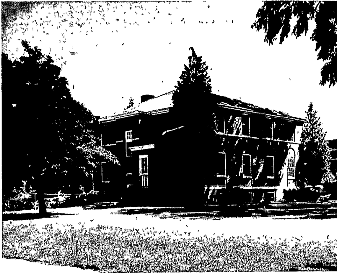
This building was formerly a nurses residence and now houses the Clinton County Mental Health Center. The building was completed in 1940 and is located on Sturgis Street.
