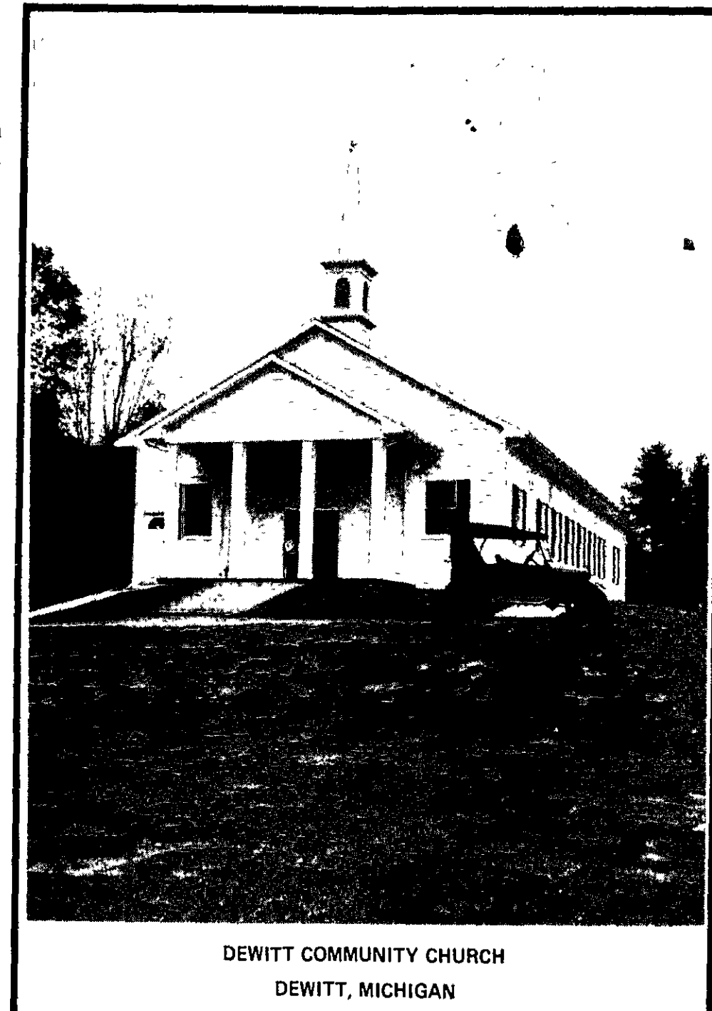
DEWITT COMMUNITY CHURCH DEWITT, MICHIGAN
