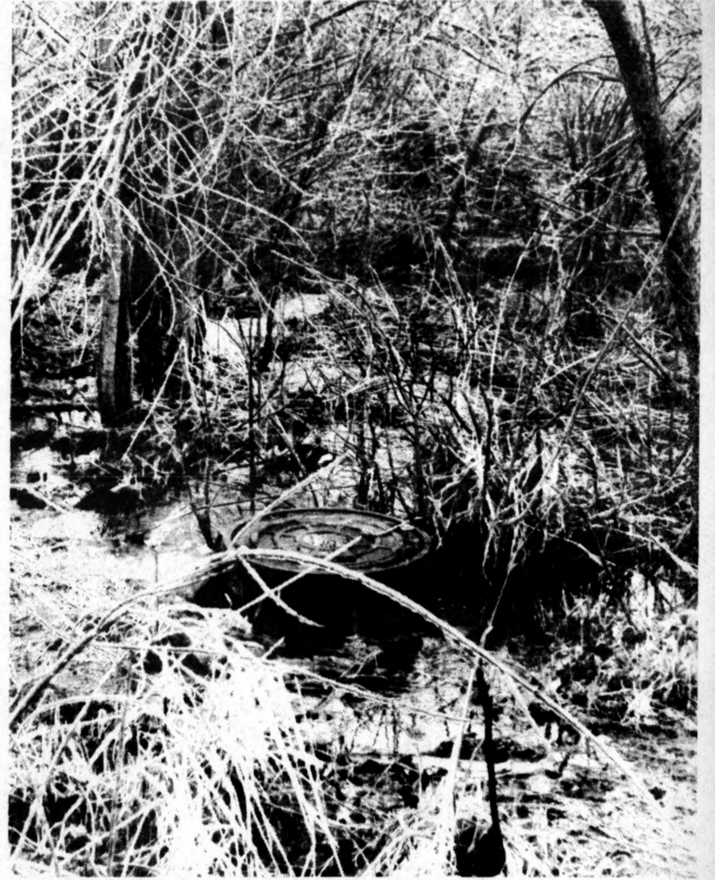
Bubbling sewage Untreated sewage flows from a manhole directly into Prairie Creek (in the background, in DeWitt Township.) The sewage is causing excessive algae growth upstream, but a waste water plant official said nothing could be done to stop the overflow. (Photo by Tom Nowak)
