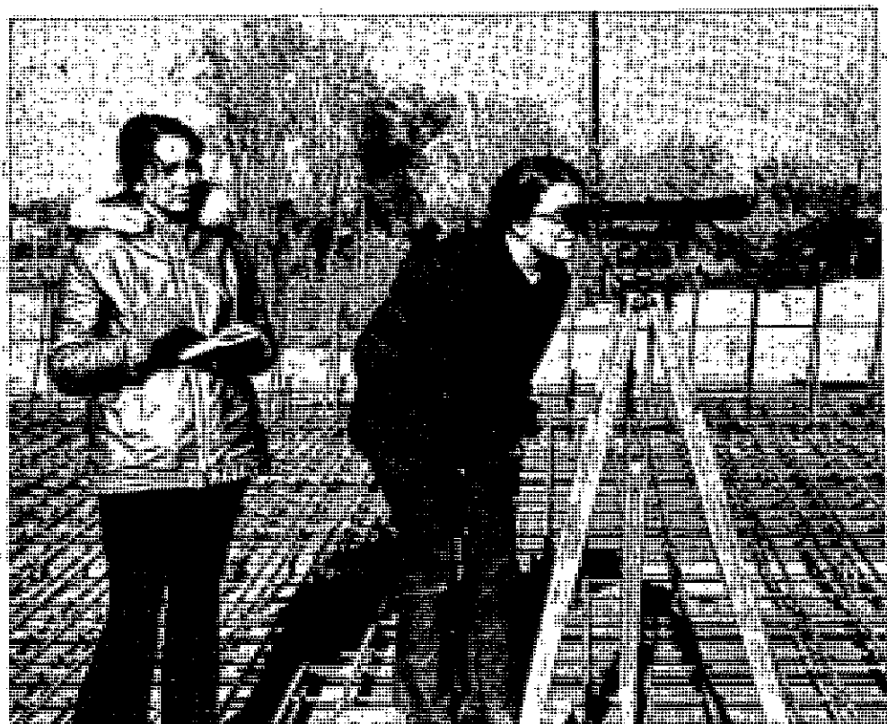
Kathy Papapanos (left), Lansing, and Marsha Walton, East Lansing, help supervise highway construction on extension of US-127 Freeway north of Lansing. They are among four female graduate engineers hired by the Department of State Highways to undergo the same trainee program their male counterparts are required to complete.
