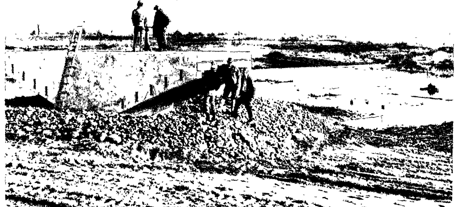
Officials of the Soil Conservation Service and the Mich Dept of Natural Resources inspect the work at the Sleeps Hollow State Park dam site now completed.
