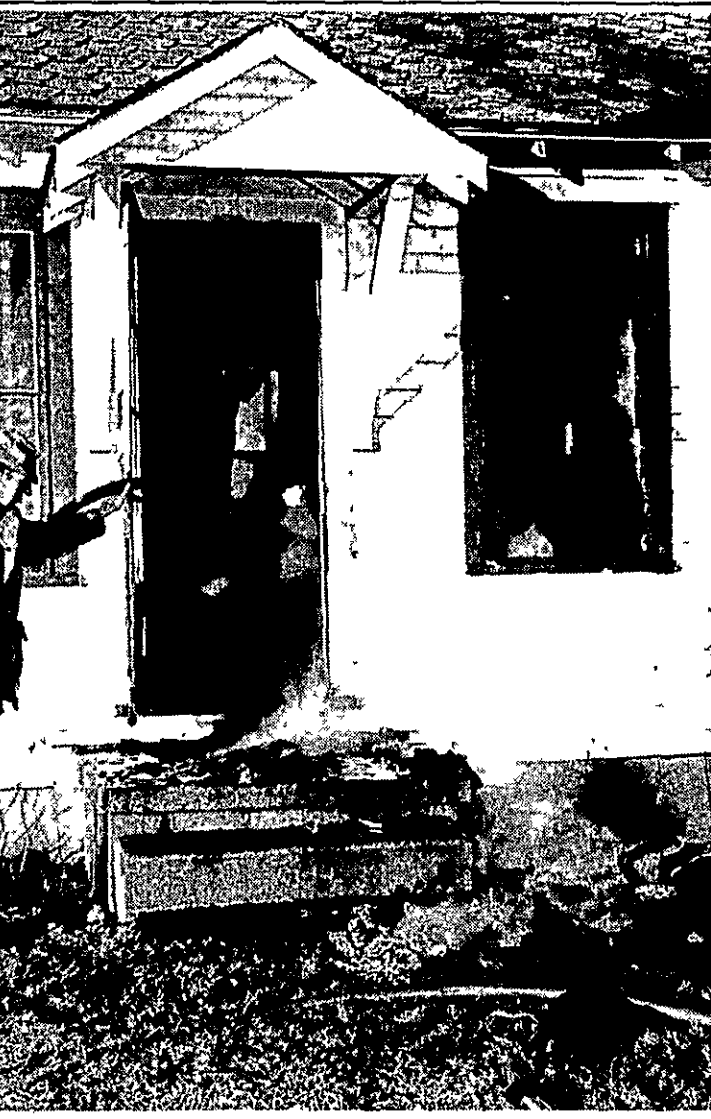
HOME DAMAGED IN FIRE
