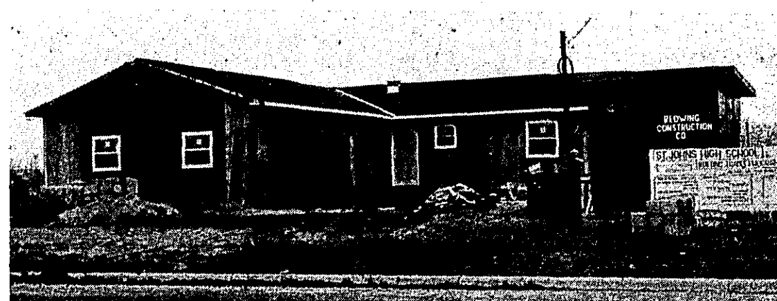
REDWING CONSTRUCTION CO.
