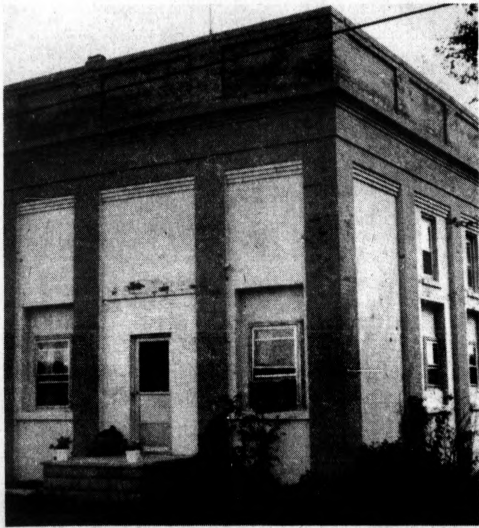
Inter-Urban power plant
