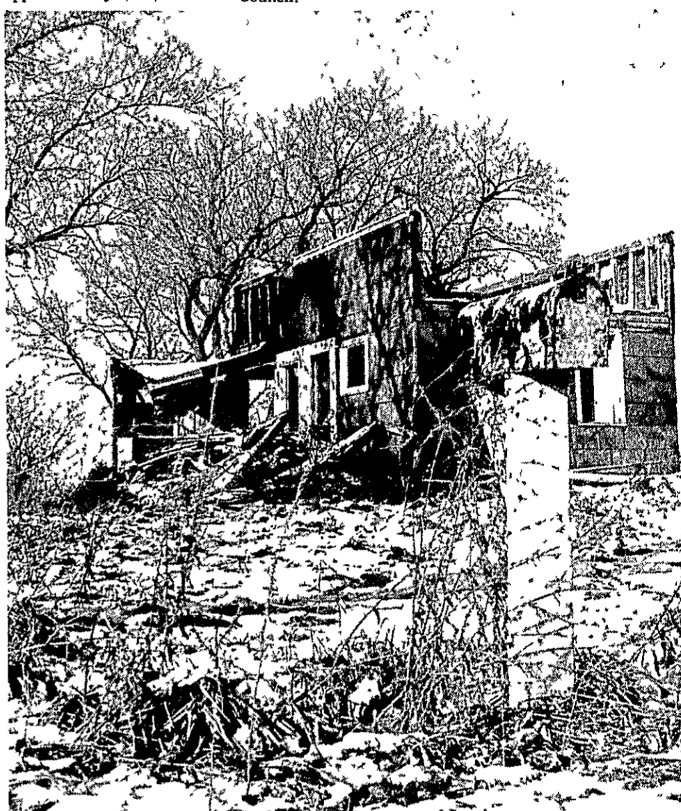
The walls haven't come tumblin' down at this house on South Townsend Rd and the neighbors don't like it. They've asked city commissioners to do something about it. St Johns Fire Chief Clare Maier reports the owners applied for a burning permit after the commission put the heat on.
