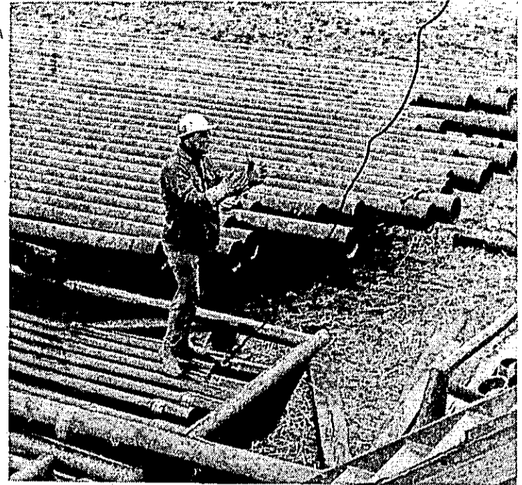
Workman ready to hookup 30-foot drill extension
