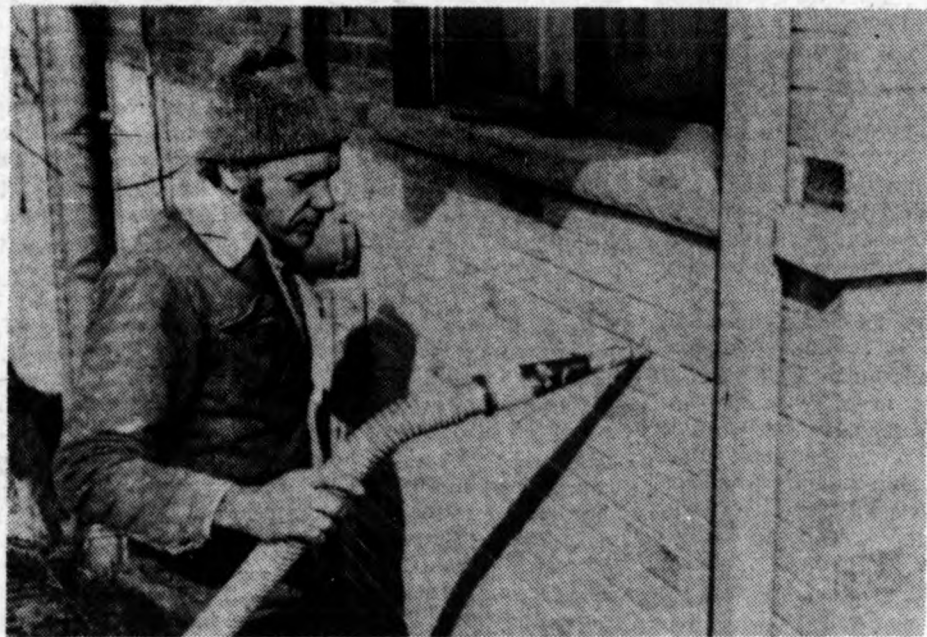
Insulation applied with blower
