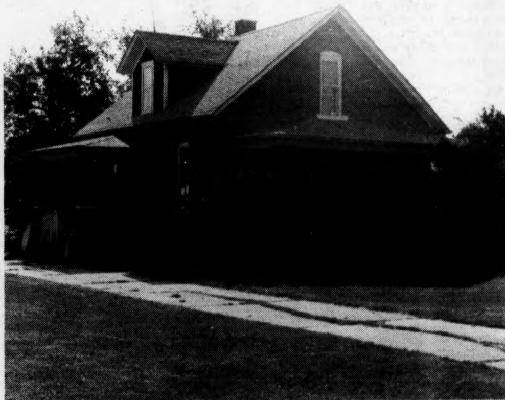
CLINTON COUNTY HISTORICAL MUSEUM VICTORIAN COTTAGE (c. 1880) 1009 S. Oakland St.
