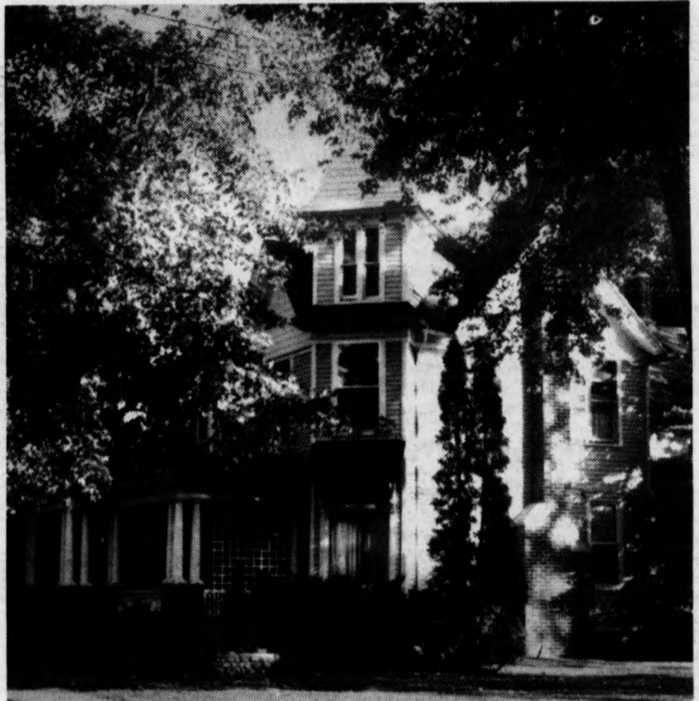
SHEAP HOUSE (Ward) - ITALIANTE (1892) 309 W. Baldwin; Residents Mr. and Mrs. Robert Sheap
