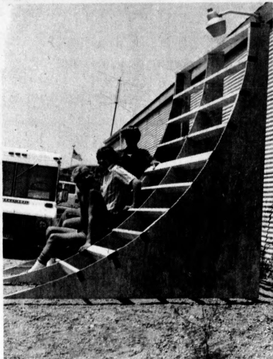
Ramp being built
