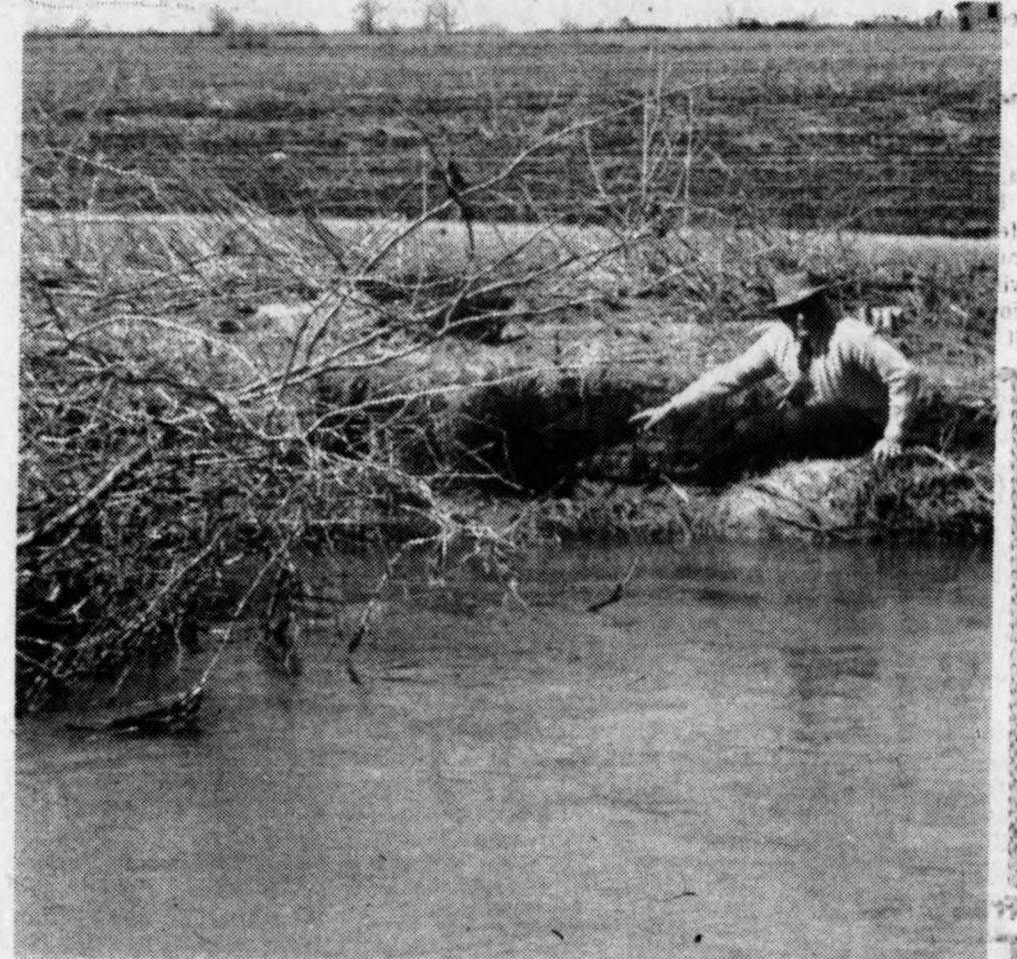
Clinton County Drain Commissioner, Harry Harden, points to erosion of the Stoney Creek banks which he says is caused by the meandering of the water. (Photo by Sue Kiley)
