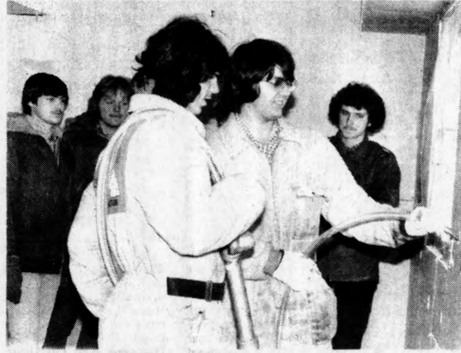
In goes the insulation
