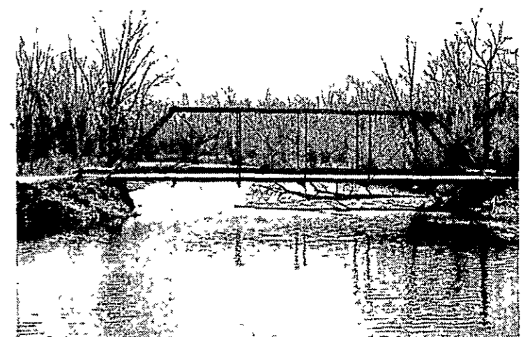
This picturesque bridge on Tallman Road will be replaced Dec. 6 with a new structure costing $234,552. Richard Waters was the contractor at that time and E. E. Vance served as supervisor.
