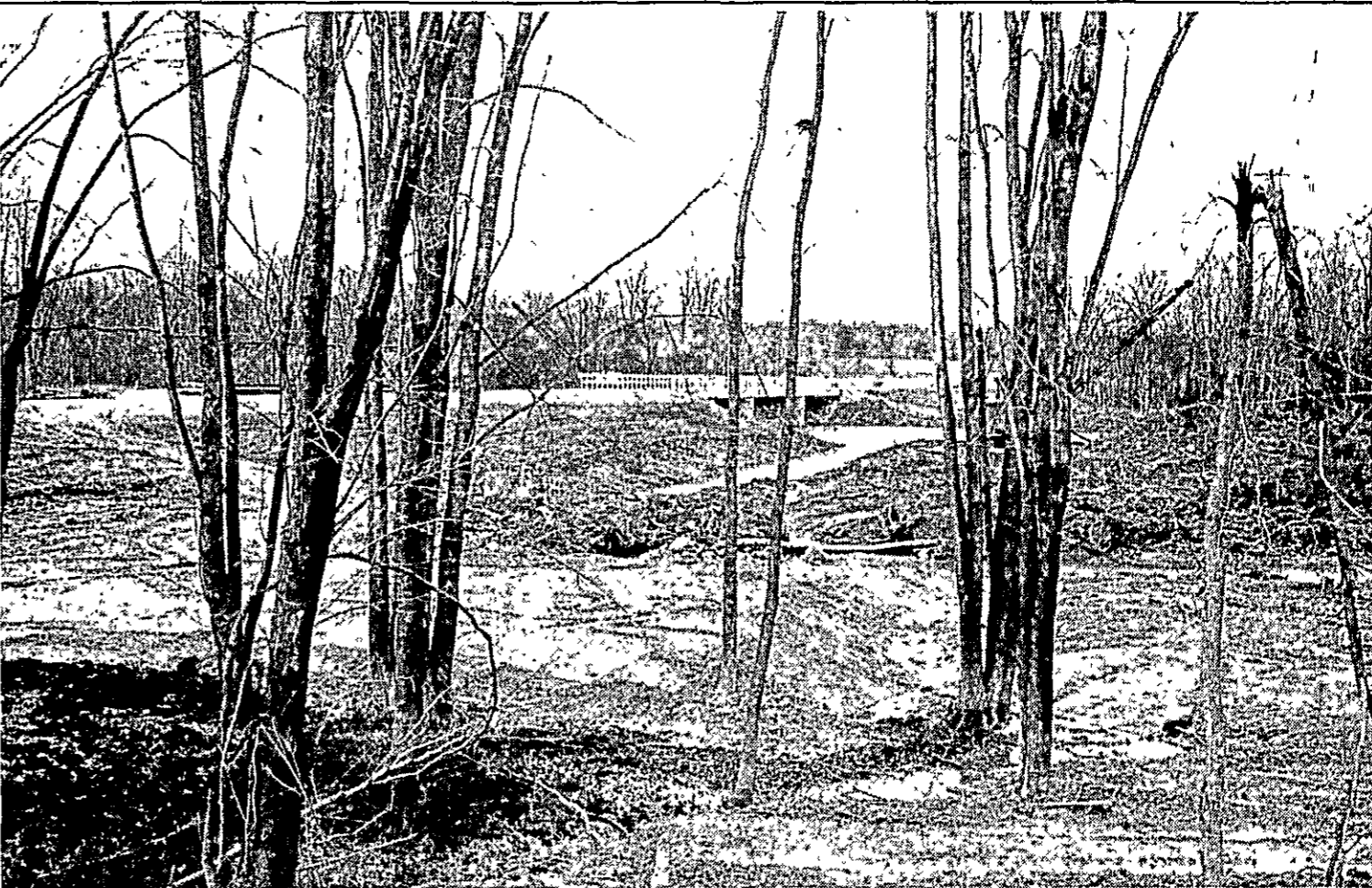
The new bridge on Tallman Road has a setting of tall trees and cool waters. Scheduled to open Dec. 6 it will be the only bridge crossing the Maple River between Maple Rapids and Hubbardston. It will also eliminate a couple of dangerous turns in the road.
