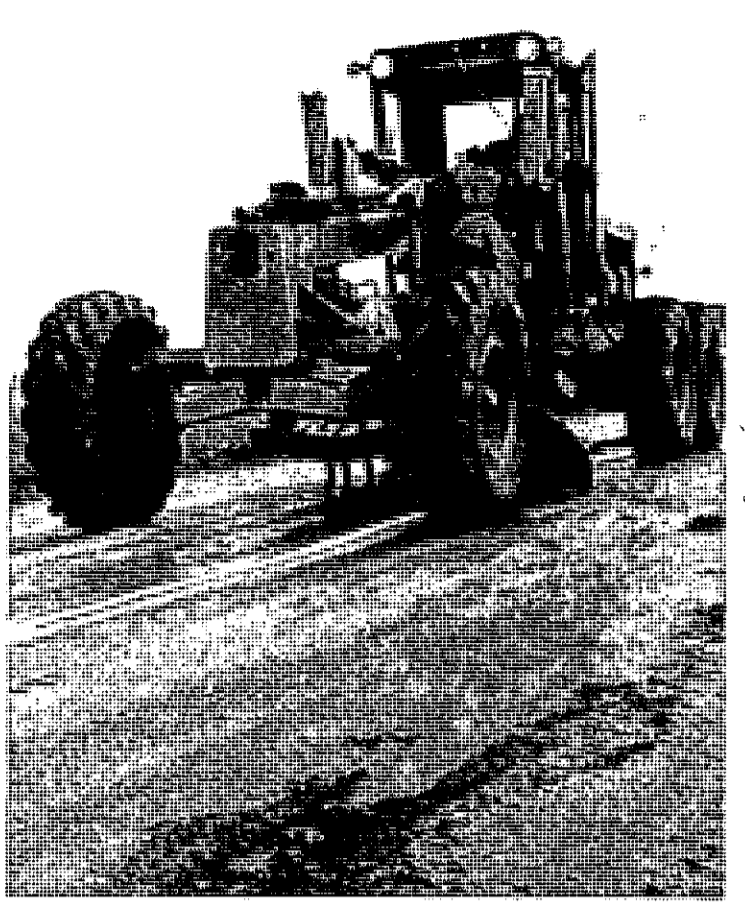
Road crews from the county road commission last Thursday roughed the surface of the section of Francis Road where several accidents have occurred in recent months. Using a road grader with a rake attachment, workmen scraped ruts in the surface layer of asphalt which has become smooth with wear.
