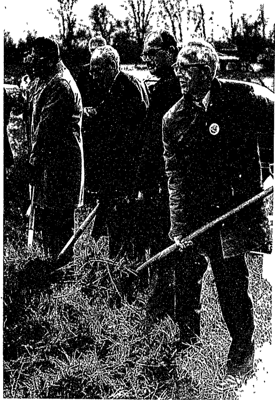
Breaking ground for the New Seventh Day Adventist Church in St. Johns are (from left) Dale Andres, contractor; Elder E. F. Herzel; Robert Wood, St. Johns mayor and Carl Mosher. Ground for the new church building on South Oakland Street was broken during ceremonies Sunday afternoon.
