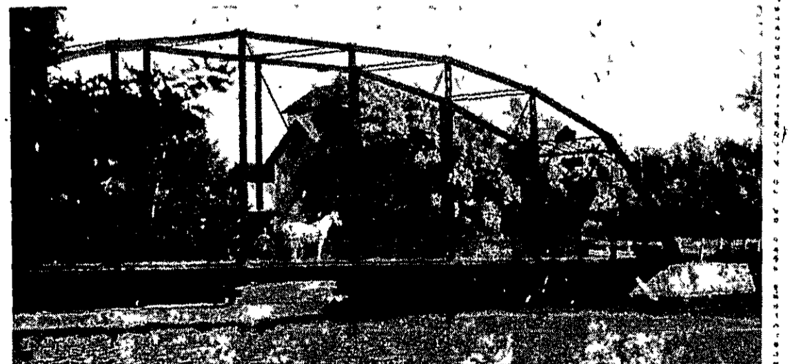
BACK IN THE EARLY DAYS OF THE ELSIE BRIDGE.
