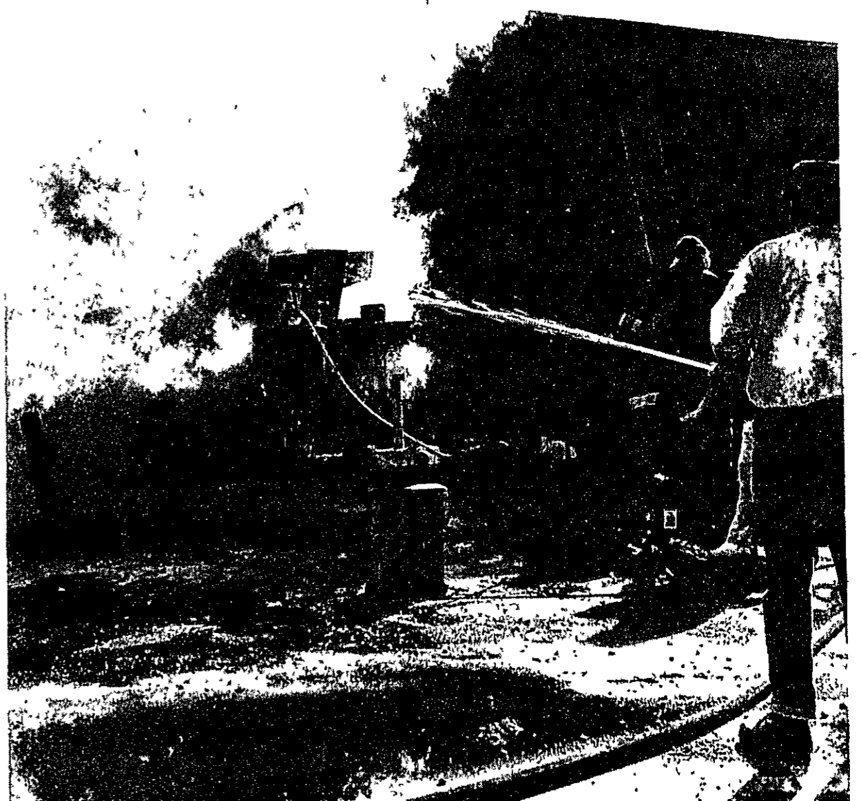
From a distance, the smoke may have made passers-by think the whole IGA Store was on fire, but it was just a roofing tar machine here being doused by St Johns firemen.
