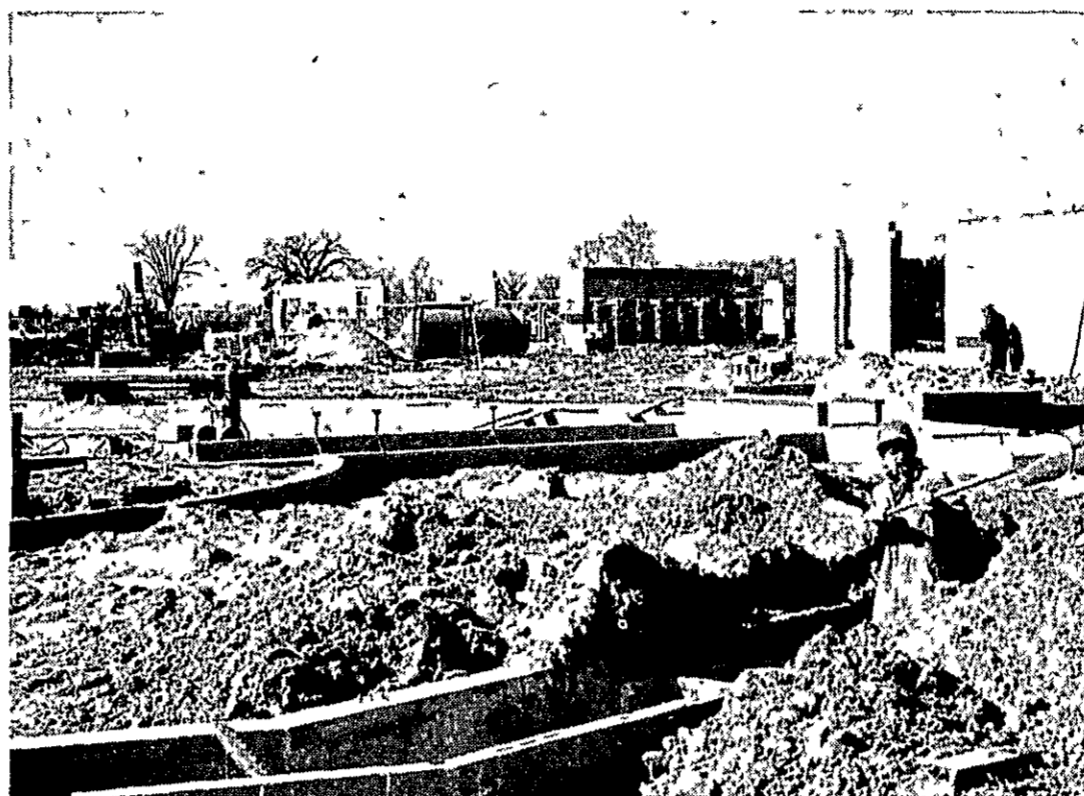
Construction worker Neil White, with the Andy J. Egan Co. (plumbing) heating and ventilating contractors, digs out a perimeter tunnel at the east edge of the new St. Johns High School science wing. The concrete floor of the wing will be poured as soon as final plans arrive and plumbing and electrical conduits can be installed. At right in background is the curving wall of the main academic cluster, while going up in the center background are walls for the home economics area.
